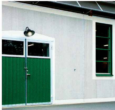
Highly insulated swing door, green lacquered profiled steel sheet, with associated thermal windows.
