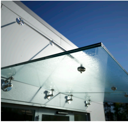
Glass entrance door.
