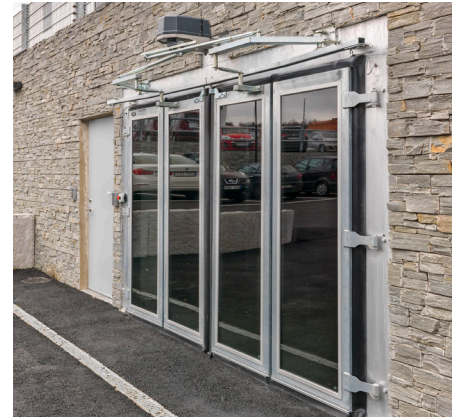
When function meets design, fully glazed doors for optimal light transmission in the car park.
