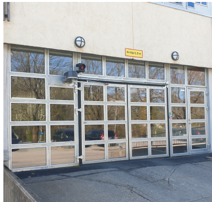
Let the light in but not the cold - Fully glazed section with machine-operated folding doors and access door.
